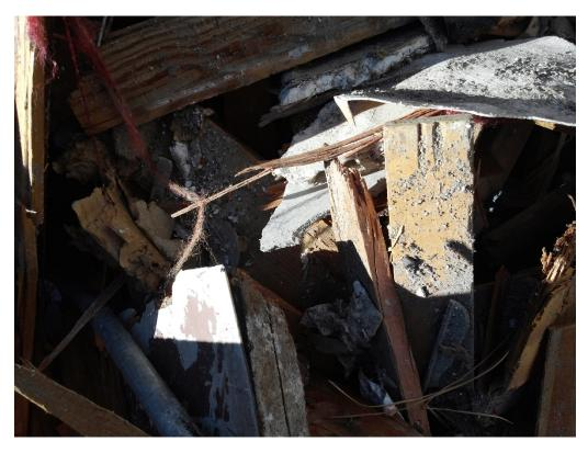
Photograph 8Date:September 25, 2019Direction: DirectImage demonstrates crumbled sections of Category II nonfriable ACM associated with the debris pile<br/>generated during the initial demolition at the Reindeer Lodge facility.Direction: Direct
