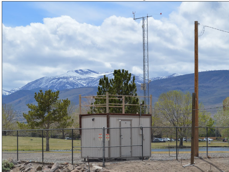
Figure 10 South Reno Monitoring Station
