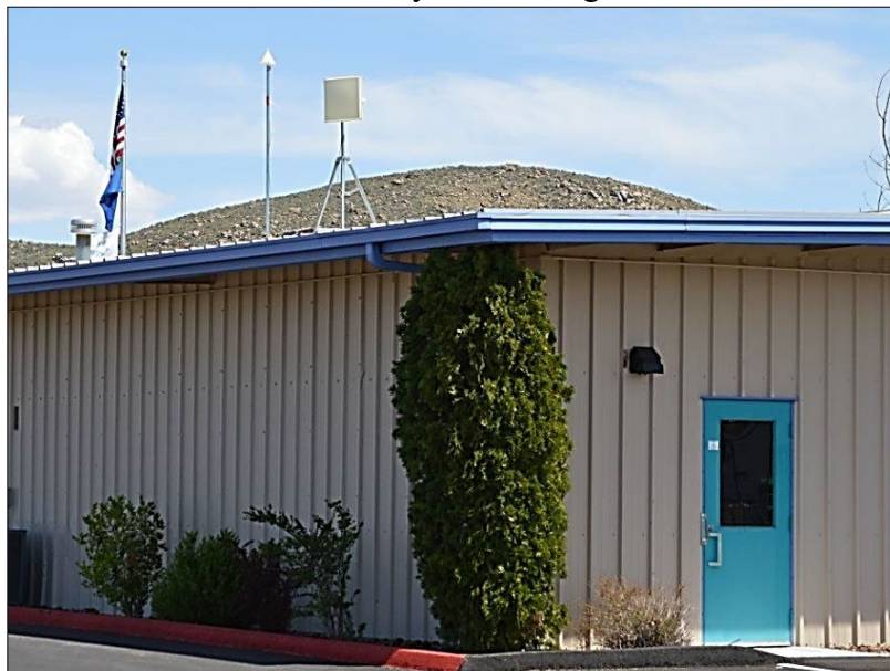
Figure 6 Lemmon Valley Monitoring Station
