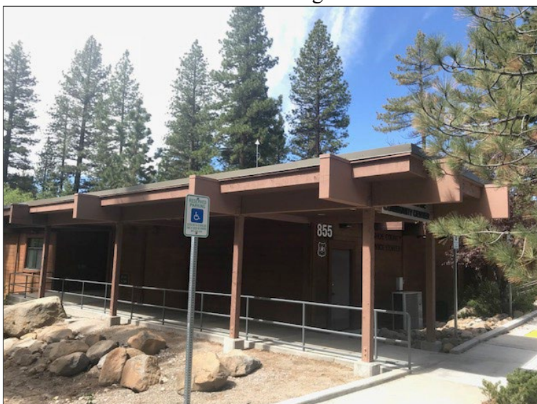
Figure 4 Incline Monitoring Station
