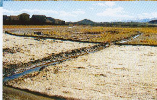
Construction of a low flow channel prevents spreading, stagnant water that breeds mosquitoes.
