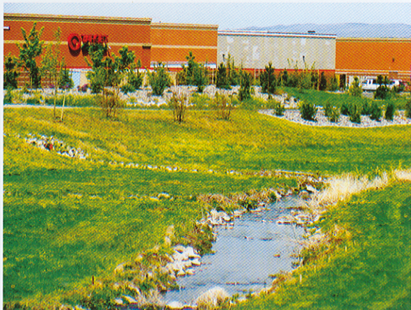
Rock-lined channels keep water moving and reduce overhanging vegetation that harbors mosquitoes.
