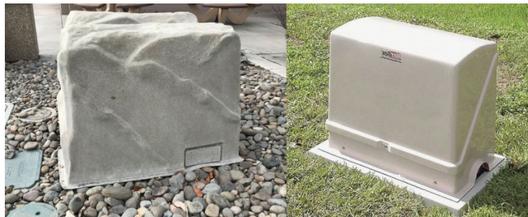
Figure 9: (Left) Hot box disguised as a rock. (Right) Typical lockable hot box.
