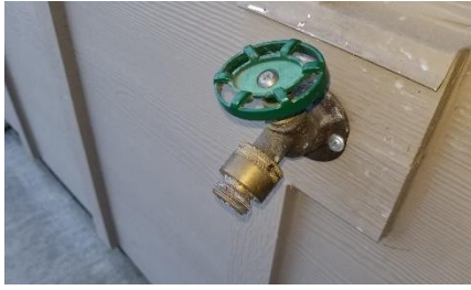
Figure 31: Hose connection vacuum breaker installed at hose bib.
