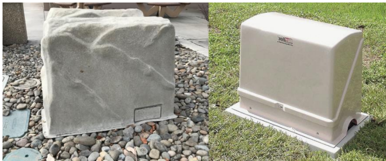
Figure 25: (Left) Hot box disguised as a rock. (Right) Typical lockable hot box.
