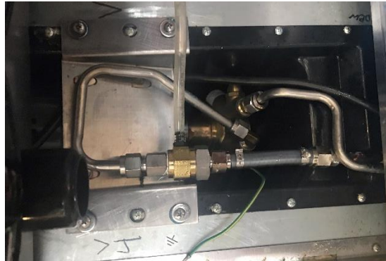
Figure 29: Dual check valve with intermediate atmospheric vent installed at beverage dispensing station.
