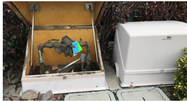
Figure 28: (Left) Typical installation of RPPA inside a food facility where piping is held 1" off wall using clear acrylic block and device has an air gap fitting installed on the drain line to ensure device is indirectly drained. (Right) RPPA installed in an outdoor hot box.
