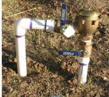
Figure 32: Pressure vacuum breaker installed on irrigation system.
