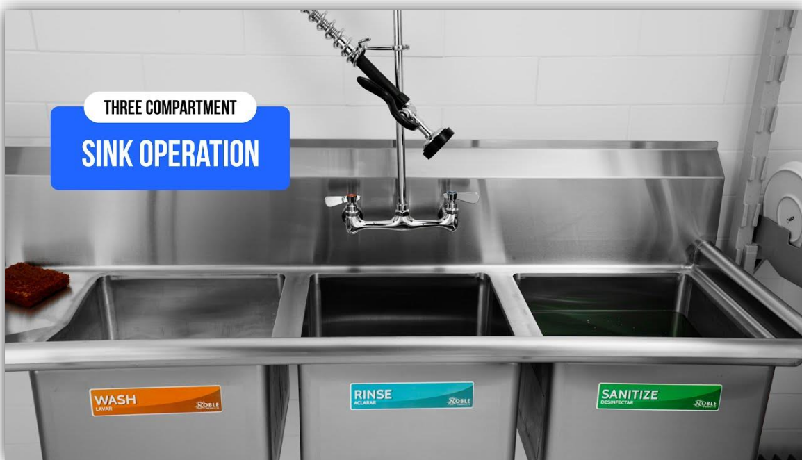
Figure 6 - Three compartment sink with proper set up
