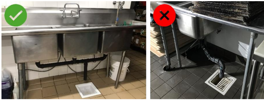
Figure 34: (Left) 3-compartment sink drain line properly air gapped to floor sink. (Right) Prep sink incorrectly plumbed with drain line below rim of floor sink.
