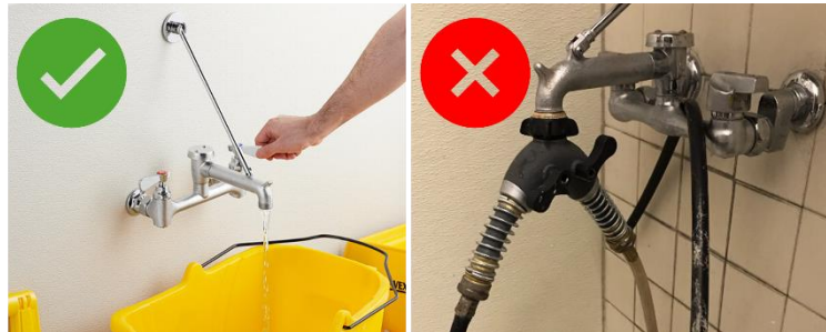
Figure 30: (Left) Properly installed atmospheric vacuum breaker on mop sink faucet. (Right) Prohibited y-valve connector installed on mop sink faucet that must be removed.
