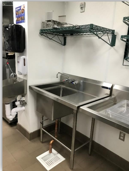
Figure 5 - Prep sink with indirect drainage
